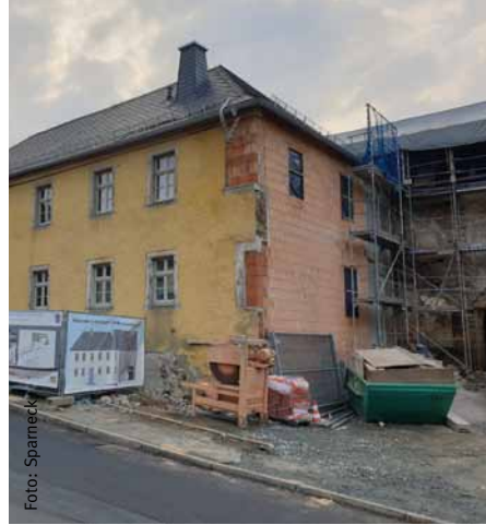
Baustelle Münchberger Straße 1 in Sparneck
